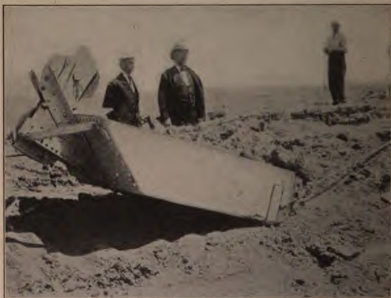
Scraper Bucket of Tower Excavator.
